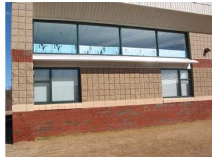
Fig. 22: Modified window configuration with opaque board
