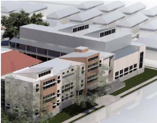
Fig. 10. Roof monitors at new addition
