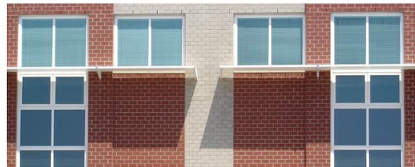
Fig. 7: Exterior light shelves with blinds between glazing
