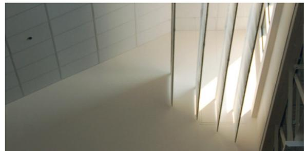
Fig. 3: Linear and ascending baffle designs in monitors
