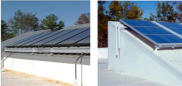
Fig. 2: Solar collectors mounted on north roof monitors
