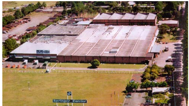
Fig. 3: Exterior Existing Conditions.
