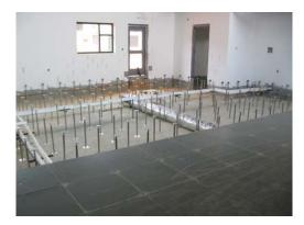
Fig. 8 Underfloor system construction
