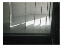
Fig. 6 Baffles in monitor well cutting off direct sunlight
